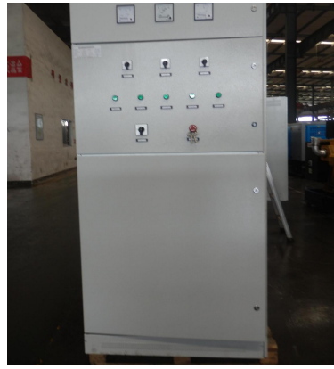
ATS (automatic transfer switch) system
